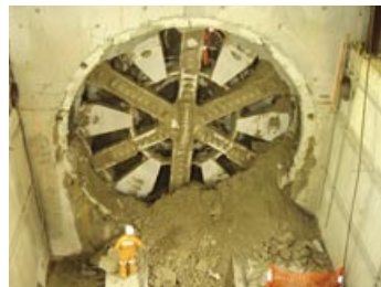
The Tunnel Boring Machine at the time of its arrival in Perth Yard.
