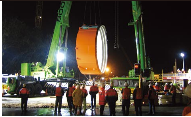
A large hole is bored at the position of the present Esplanade Station. From there the components of the Tunnel Boring Machine are brought in.
